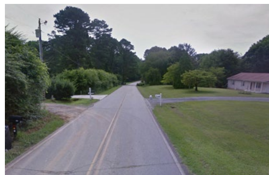
Existing Thompson Creek Park Rd.
