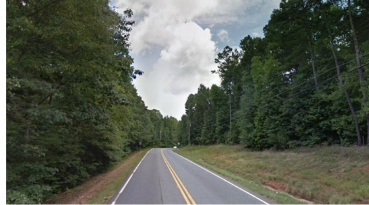
EXISTING HIGHWAY 53 NORTH
