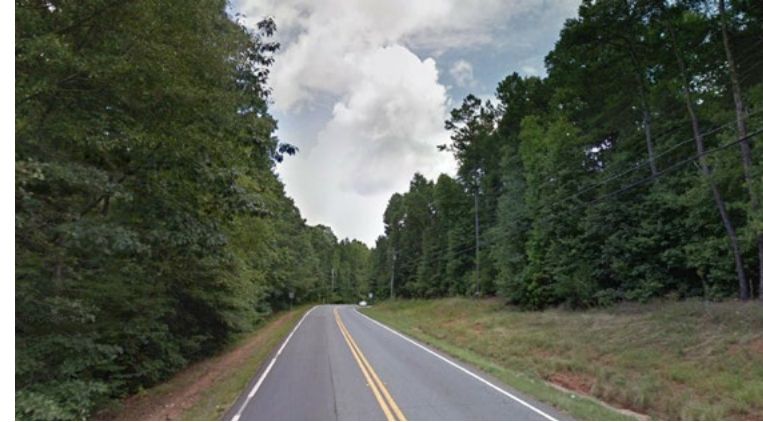
EXISTING HIGHWAY 53 NORTH
