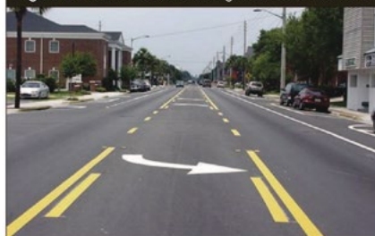
Figure 2. Photo. Three-lane configuration after road diet.
